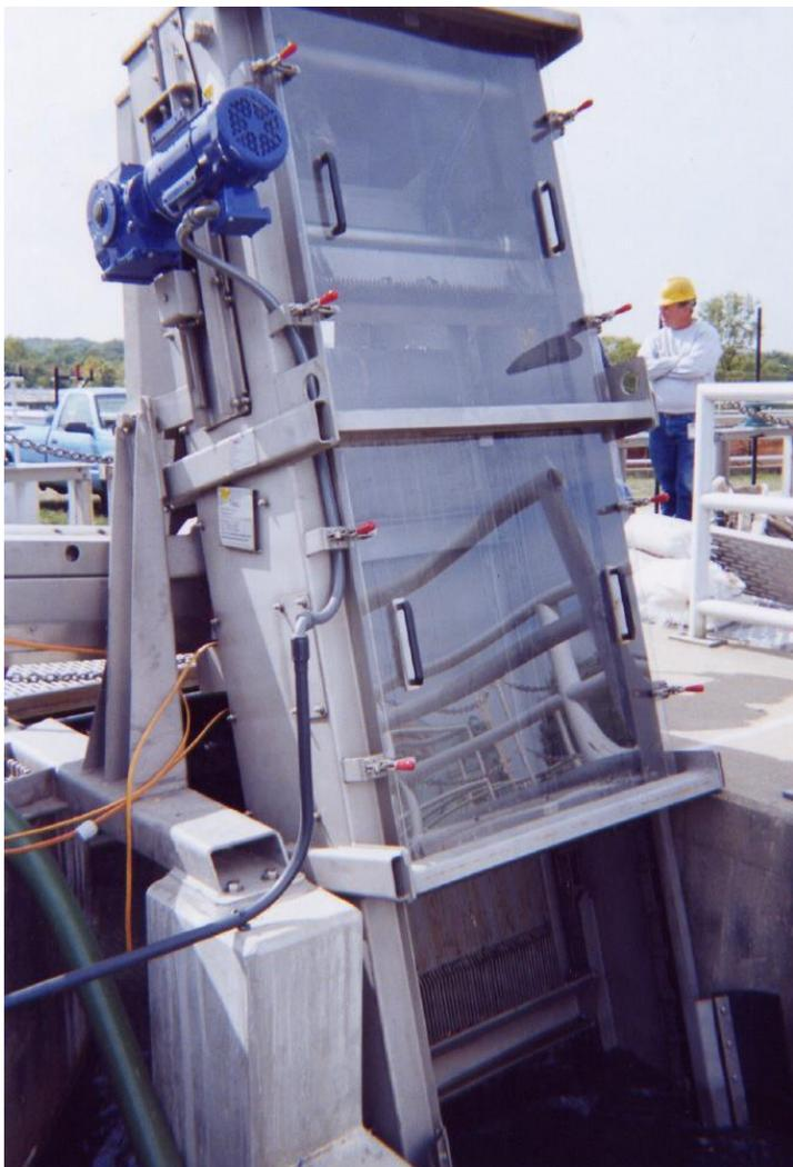
The primary treatment process consists of the removal of sand, grit and large solids and is an important first step as it can remove 45-50% of the pollutants. If the equipment for this part of the system is not effective, then the rest of the plant will not function well. Understanding the importance of superior quality and reliability in the primary treatment processes, the WSSC contacted Headworks® to discuss Piscataway's screening equipment needs.
