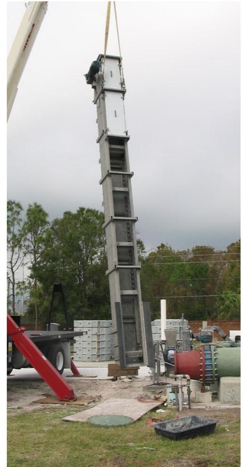
*Due to space constraints both screens were removed from the channel individually to execute the retrofit*
