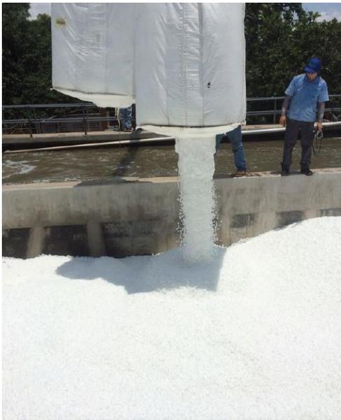
*ActiveCell media increases productivity through providing protected surface area to support growth of bacteria.*
